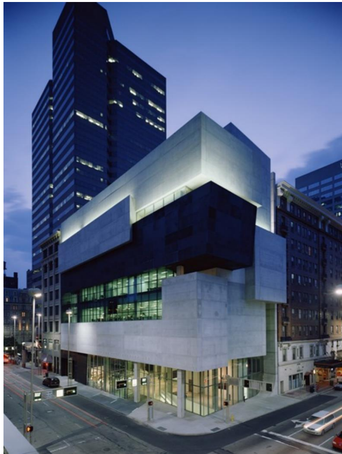
Figure 1: Lois and Richard Rosenthal Center for Contemporary Arts (Southeast Exterior)
